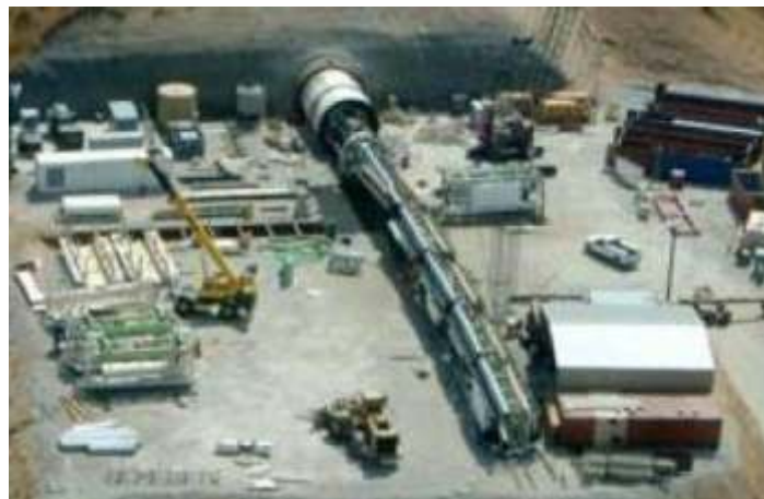
The envisaged tunnel machine to excavate a 14km tunnel at Murrurundi
